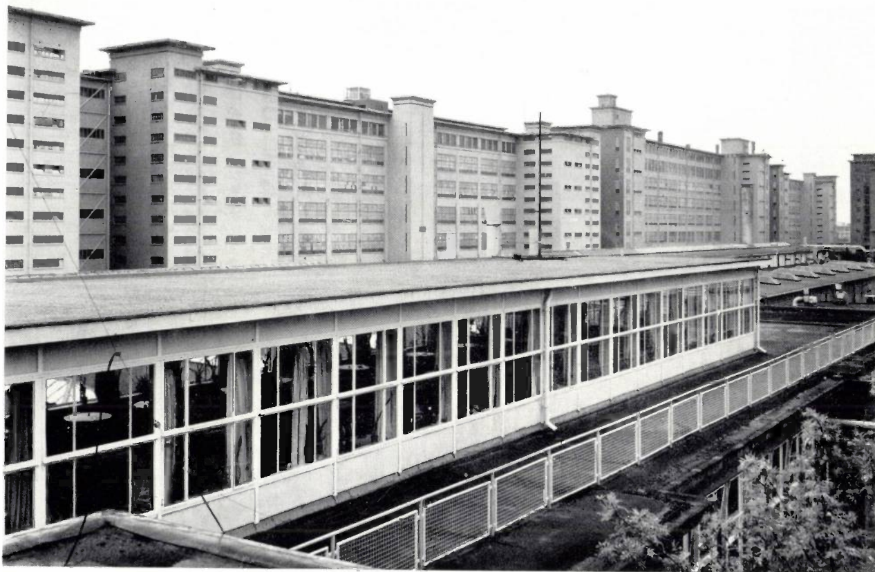
Fig. 14. Glass wall of a canteen on the roof of the Research Laboratories and the roof balustrade 3 m in front of it, each separately visible in the radar display in fig. 13 (marked by arrow). The tall factory buildings in the background can be seen top left on the radar screen.
